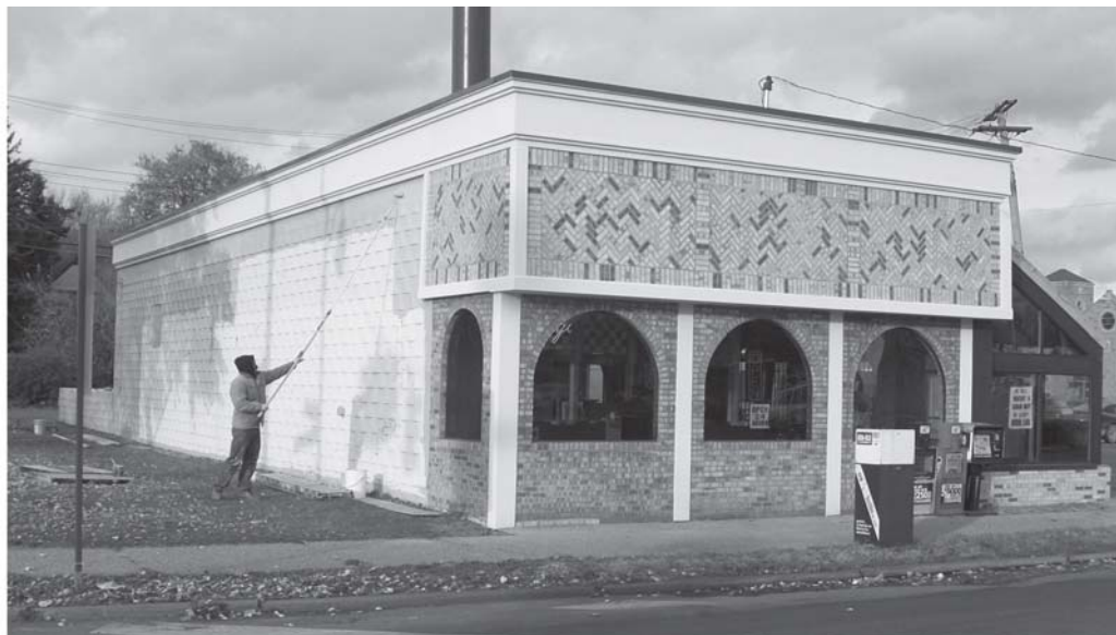
Worker applies paint to the masonry walls of the building; a new roof over the greenhouse and new signage will complete the facade improvements.
